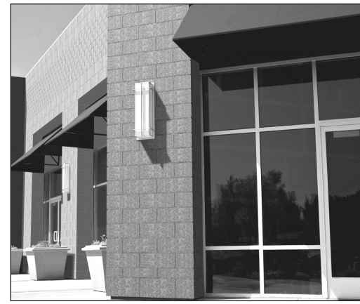
This rendering illustrates how Integrity Blocks could replace conventional concrete masonry units, or CMUs.
